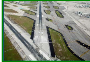
Miami International Airport Runway Rehabilitation
