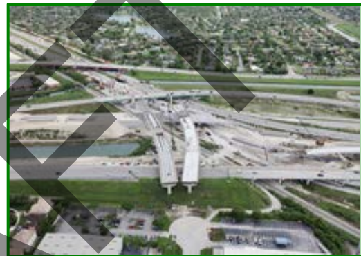
SW 128TH STREET APPROACHING SR 874 RAMP CONNECTOR
